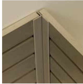
Attach Flat to panel with the edge against the Small L.
